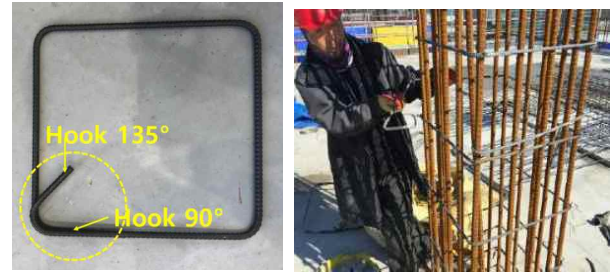
(a) Preprocessed tie bar (b) General hoops installation
