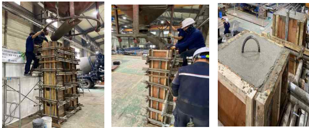
(a) Ready-mixed concrete filling
