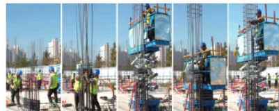
b) Method for fitting in the column top
